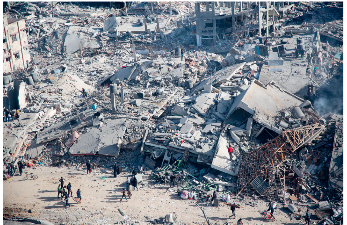
Fig. 1. Aerial view of damage around the Al-Shifa Hospital, Gaza City, Palestine. April 1, 2024
