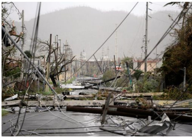
Fig. 2 A damaged road west of San Juan after Hurricane Maria, September 2017
